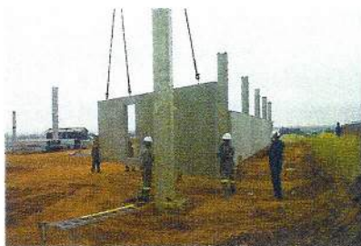
Tilt-up construction removes the possibility of mistakes and avoids the process of continuously mixing concrete on site
